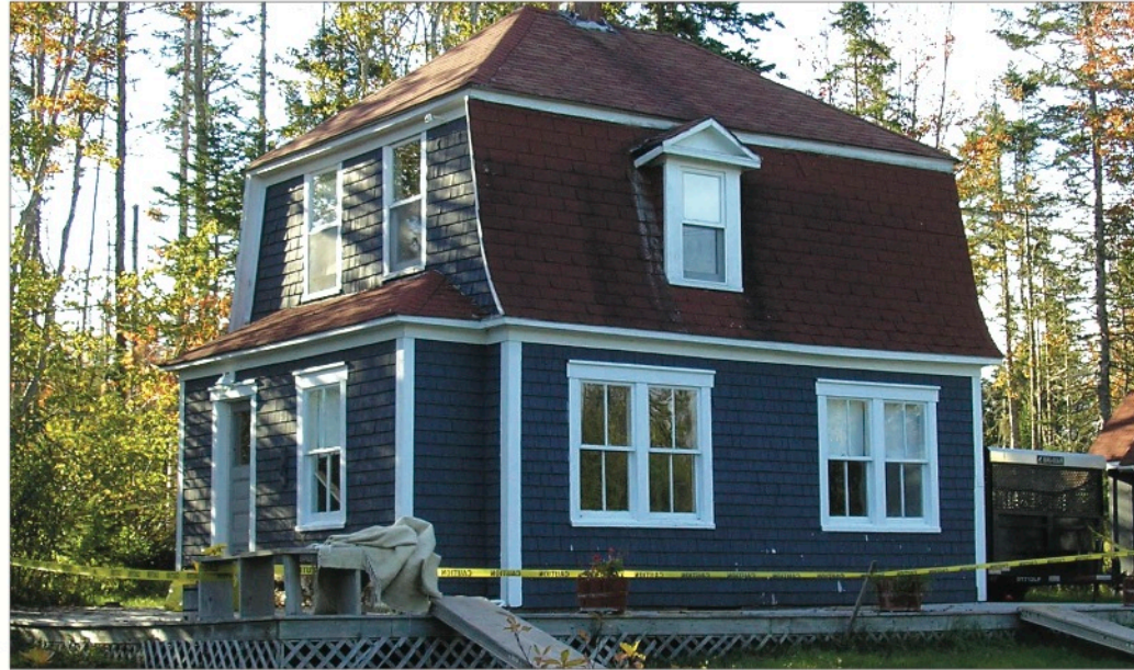
Former Matheson House - Crescent Grove, Baddeck Bay
