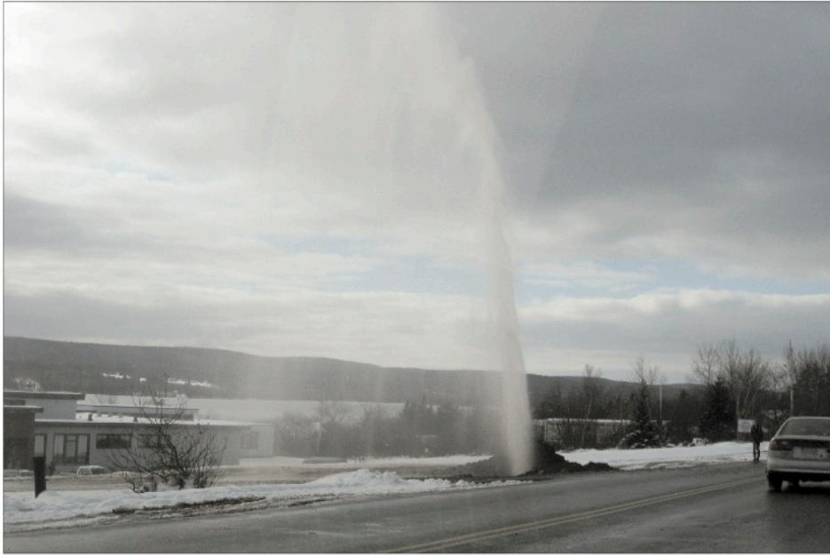
During the process of turning off the water main at Baddeck Academy, the shut-off valve plate sheered its bolts. Fortunately, neither the wrench which was torn from his hands nor the gusher of water hit Public Works Manager, Ron McIntyre. Students at Baddeck Academy also considered themselves fortunate when classes were cancelled for the day while repairs took place.
