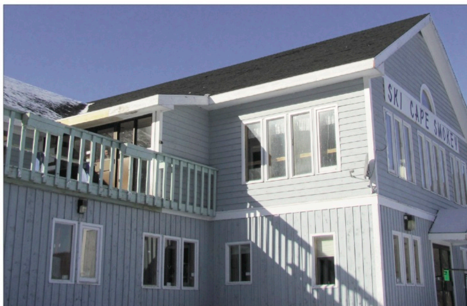
The Lodge at Ski Cape Smokey sports a repaired and reshingled roof thanks to the building's owner, the Province of Nova Scotia.
